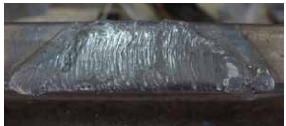
P2 for plain rail defects
