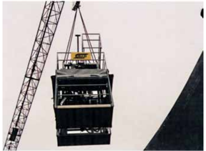
Double-side Circotech being lifted onto the job.
