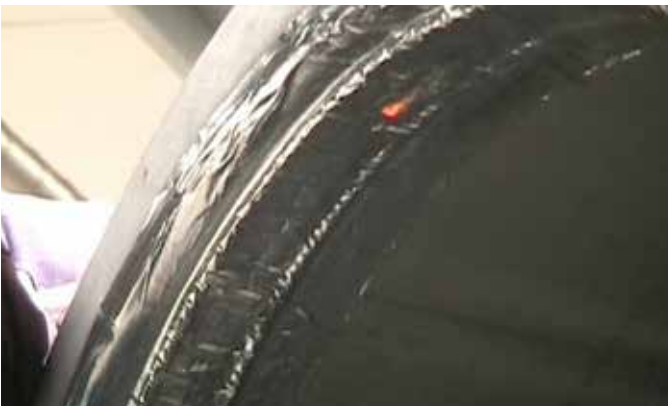
Step 2: Weld onto the Argweld® Purge Tape ®
